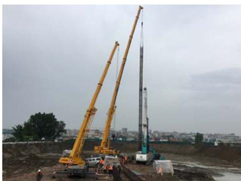
Cage placement with O-Cell assembly for TP02
