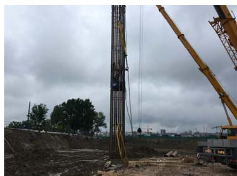
Cage placement with O-Cell assembly for TP01
